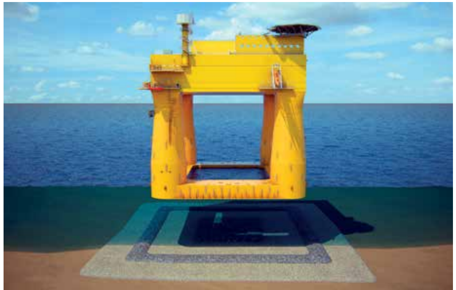
The two converter stations to be located in the German sector of the North Sea will provide grid connection for the offshore wind power plants to transmit and supply electricity to approximately a million households in Germany
